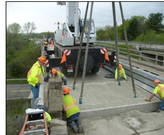
Placing panels In One Lane
