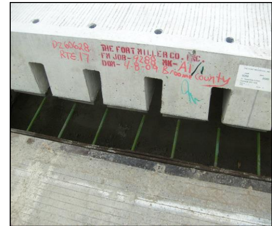
Placing panel Over Anchor Rods
